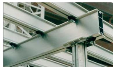
**Headplate to beam fixing**
